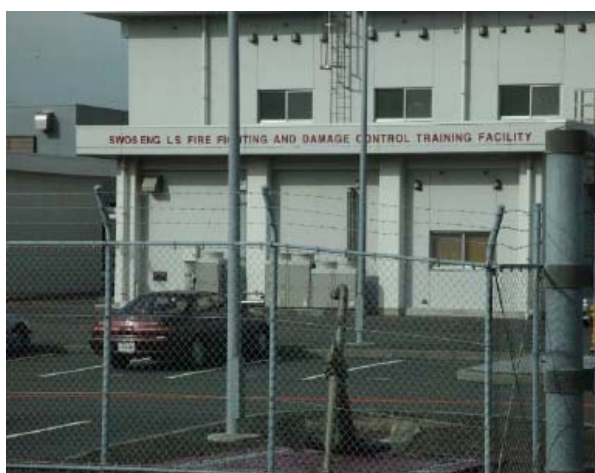
SWOS ENG LS FIRE FIGHTING AND DAMAGE CONTROL TRAINING FACILITY
